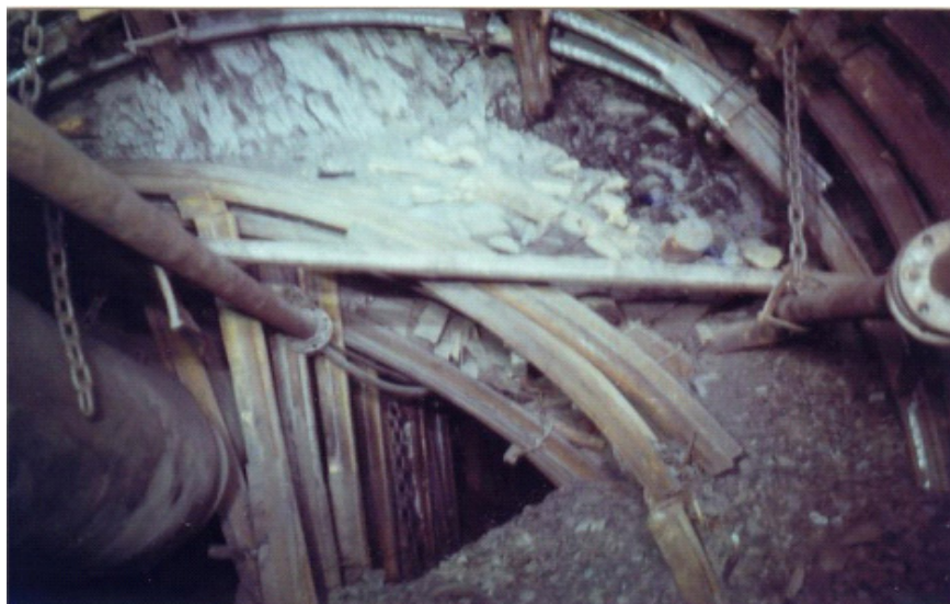
Fig. 5: Arch timbering conveyer drift state without strengthening timbering implementation ove working retimbering behind the 2nd western lava face, distance - 220 m
