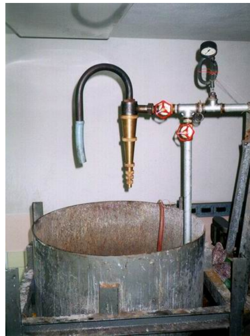
Fig. 4: Hydrocyclone station Obr. 4: Hydrocyclonová stanice
