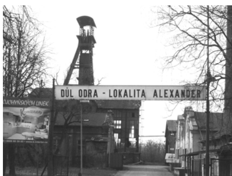
Figure 10: Alexander Mine shaft frame
