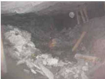
Fig. 14 Larger event magnitude ejects rock even into the gully (note dislodged support units as a result of thrown rocks)
