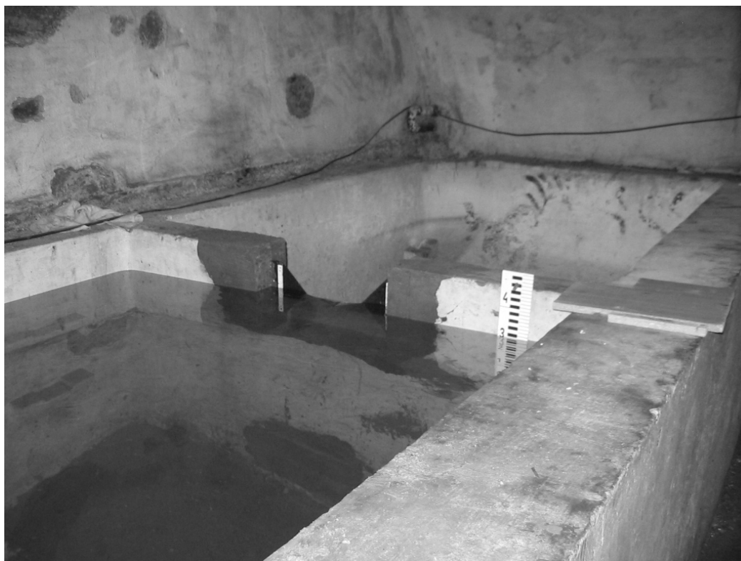
Photo 2: Disposal basin for water consumed by heat pump
