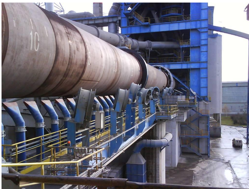
Fig. 1 Rotary kiln for cement production
