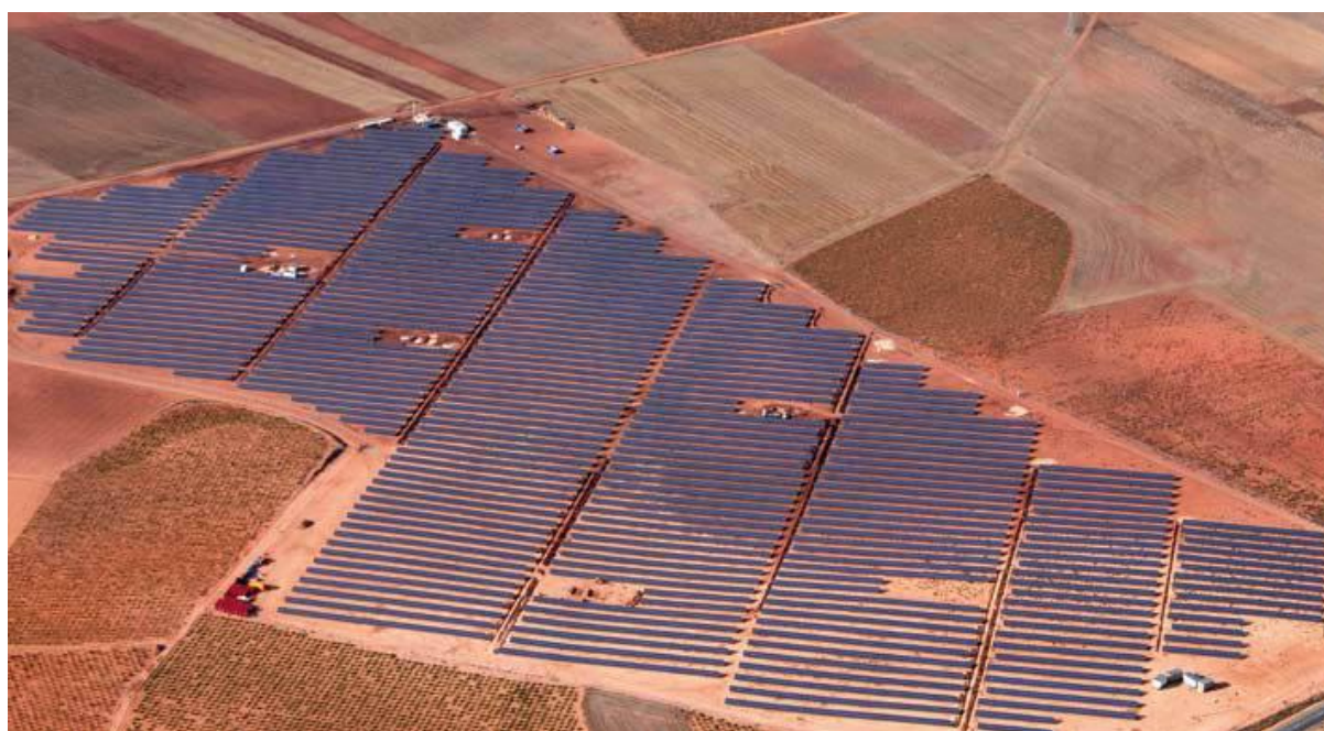
Fig. 3 Photovoltaic power plant, having an installed capacity of 6.5 MW in La Solana (Spain) [8]
