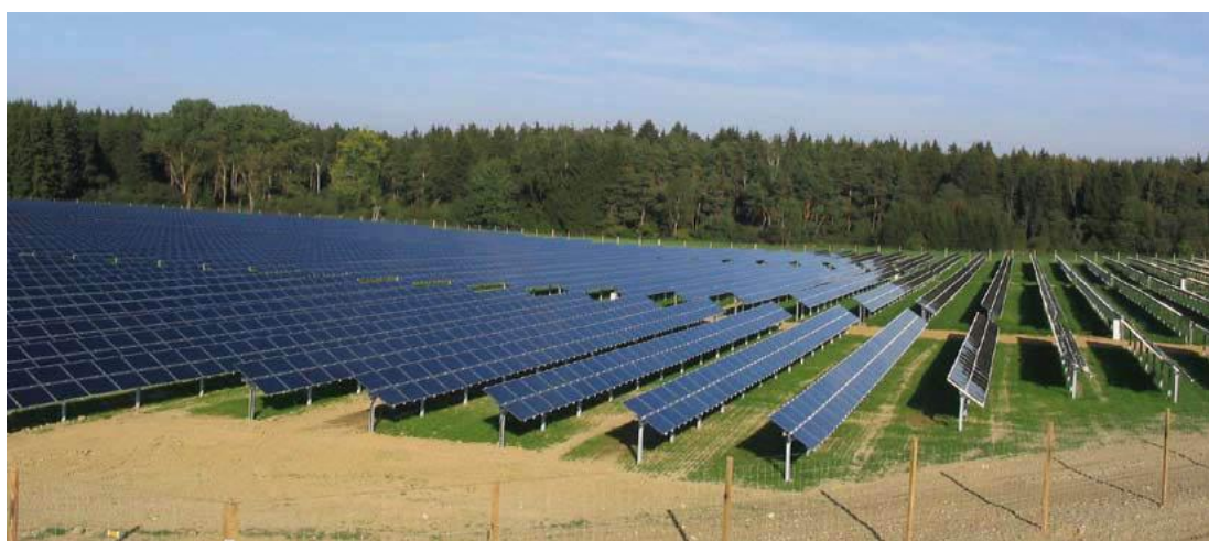
Fig. 2 Photovoltaic power plant with an installed electric output of 2.2MW in Althegenberg (Ger.) [8]
