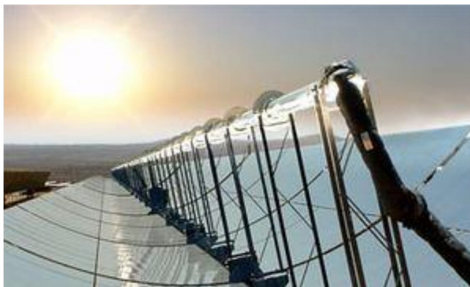
Fig.1 Parabolic mirrors and glass absorbers [ 4]
