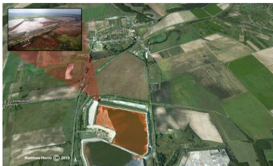
Pic. 2 Dykes accident in Kolontár
