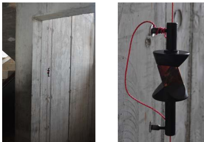
Fig. 9 360° mini-reflector Leica GRZ 101 fixed on plummet hanging
