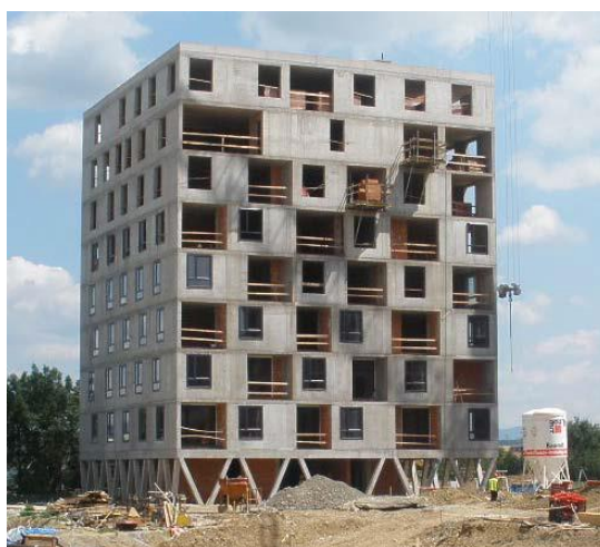
Fig. 1 SO - 03 Dwelling house HB3 at the construction of “Košice bývanie -1.etapa”
