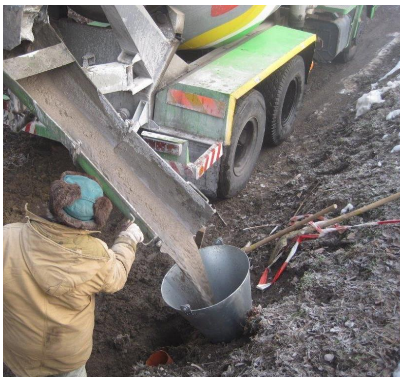
Fig. 2 Closing old mine (the photo taken by UNIGEO, a.s.)
